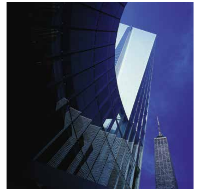
Exterior, Sofitel Chicago Water Tower, Chicago, USA
